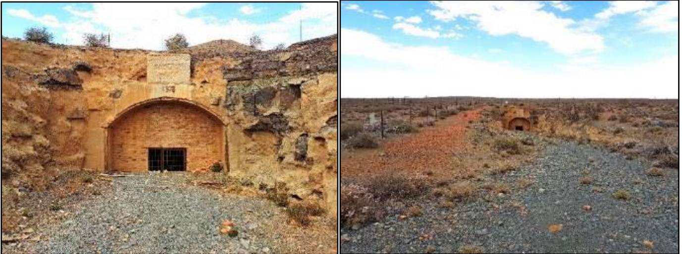
Figure 10: Trial Mine Decline Entrance on the Ryst Kuil Prospect
