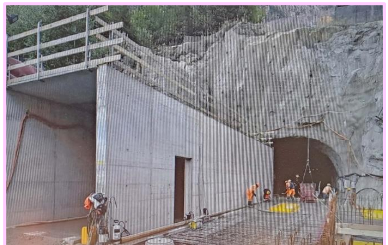
Figure 8: The New Gottard Road Tunnel (copied from Wilson, 2023)
