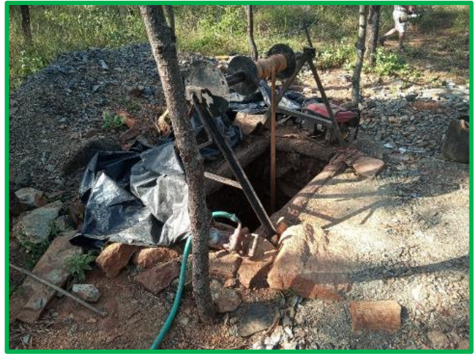
Figure 7: Shaft in the Arcturus Mine Area
