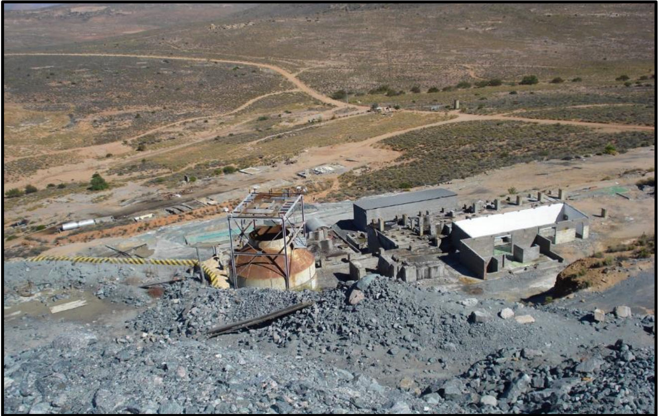
The former copper mine at Nigramoep, Namaqualand. Photo: Jo Wicht 2007
