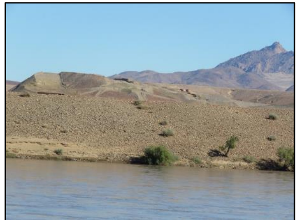
Figure 3: Detail of Berm and Spoil Mounds
